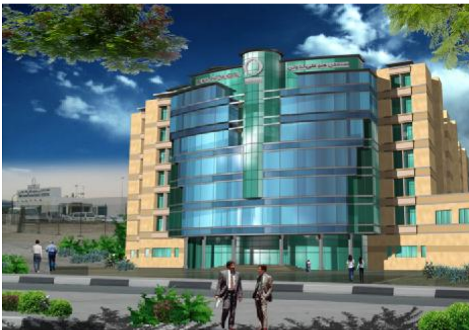
Extension building of CEDARS Jebel Ali International Hospital currently under construction
